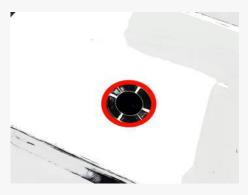
3. Drop in the waste and run a small bead around the edge of waste and basin.
